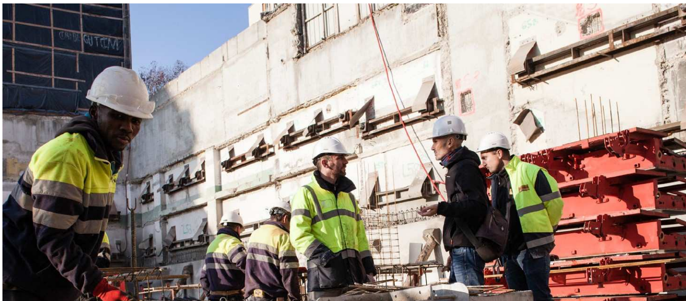
Inspection of a construction site in the département of the Hauts-de-Seine
